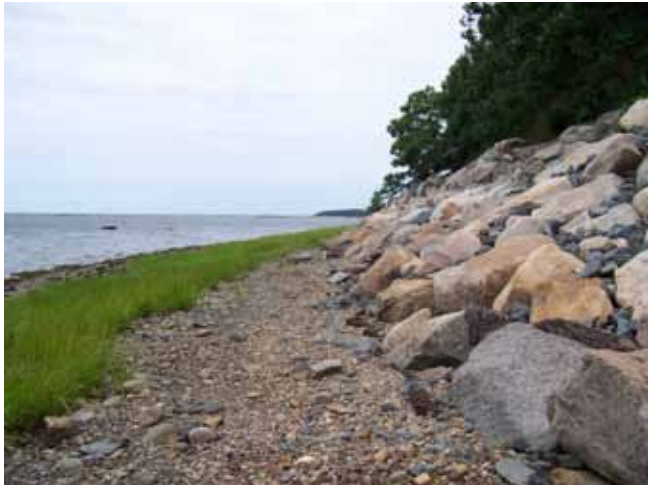
A small stony beach at the base of this rock revetment leaves little adjacent sediment supply to fronting fringe marsh. Photo: Kristen Andres.
