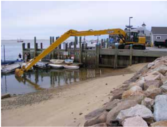
Dredging with an excavator at the Fish Pier. Photo: Ted Keon
