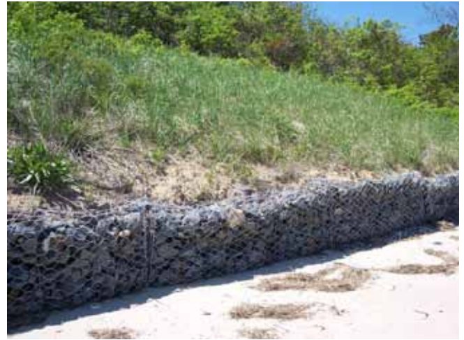
Gabions (wire boxes filled with rocks) can absorb wave energy and allow water to penetrate. Photo: Kristin Andres
