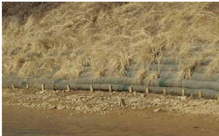
Fiber rolls, considered a "soft solution," can be covered over with vegetation to restore a natural appearance and functioning of a coastal bank. Photo: Kristin Andres
