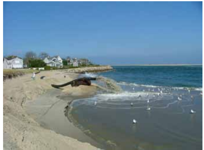
Dredged material from Aunt Lydia's Cove is pumped onto Andrew Harding Beach. Photo: Ted Keon
