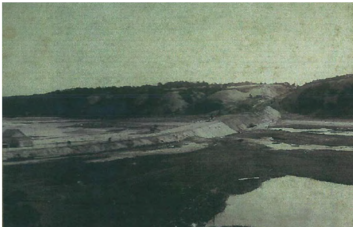
Figure 16 – Embankment Construction across Muddy Creek Estuary (c. 1900)
