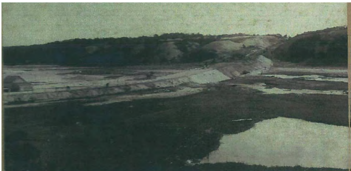
Figure 5 – Historic Photo of Earthen Fill Placement at Orleans Road (Route 28) over Muddy Creek Facing South Toward Chatham, circa 1900
