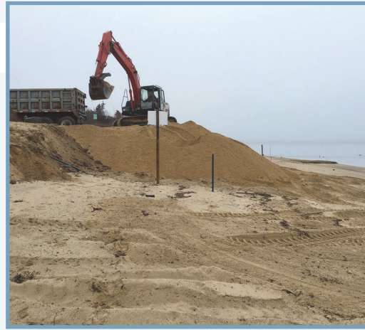
Example of proactive placement of sacrificial sand to protect upland
