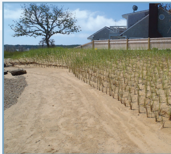
Example of artificial dune stabilized with beach grass, shortly after planting
