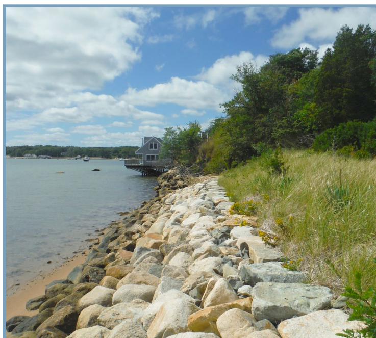
Typical rock revetment along coastal bank
