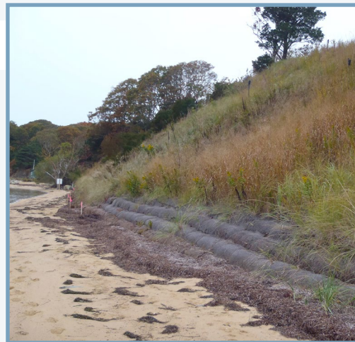
Fiber rolls used to stabilize toe of re-vegetated bank
