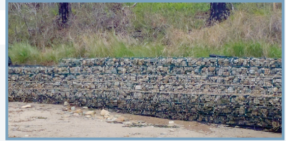
Use of gabions as toe protection
