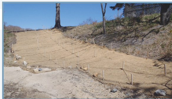
Natural jute fiber blanket to stabilize soil prior to vegetative plantings
