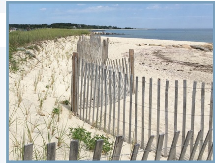
A season after fence installation, accumulated sand is planted with beach grass
