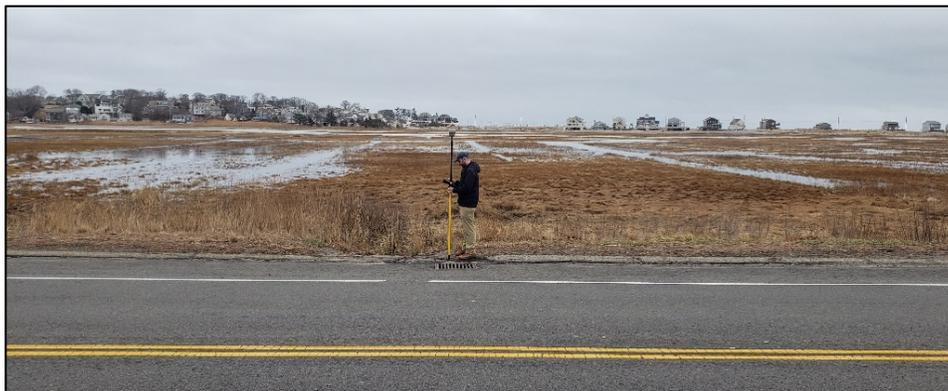
Figure 5. Example of Road STP located along an area of little relief. Water will flow from the salt marsh over the road and back into the salt marsh on the other side of the road. This image was captured in Scituate, MA (taken from Borrelli, et al., 2020).
