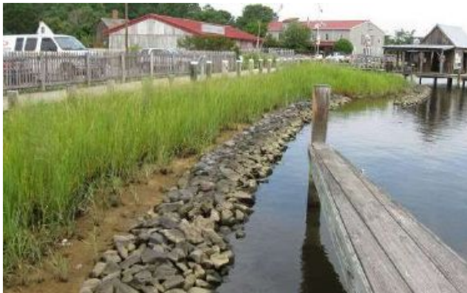
Figure 4.2 A low rock sill fronting a salt marsh restoration constructed along the eastern shore of Maryland using NOAA grant funding (Photo Credit: Chesapeake Bay Trust and NOAA).
