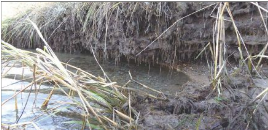
Figure 3.5 Detailed perspective of the peat bank undercutting along the tidal channel on November 10, 2020.
